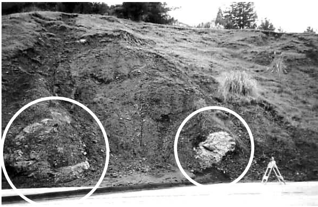
Fig. 1: Part of toe of landslide, showing typical appearance of a Franciscan Complex melange. White circles indicate large blocks of competent rock within soil-like sheared shale. Blocks shown here buttress the slopes above them.
